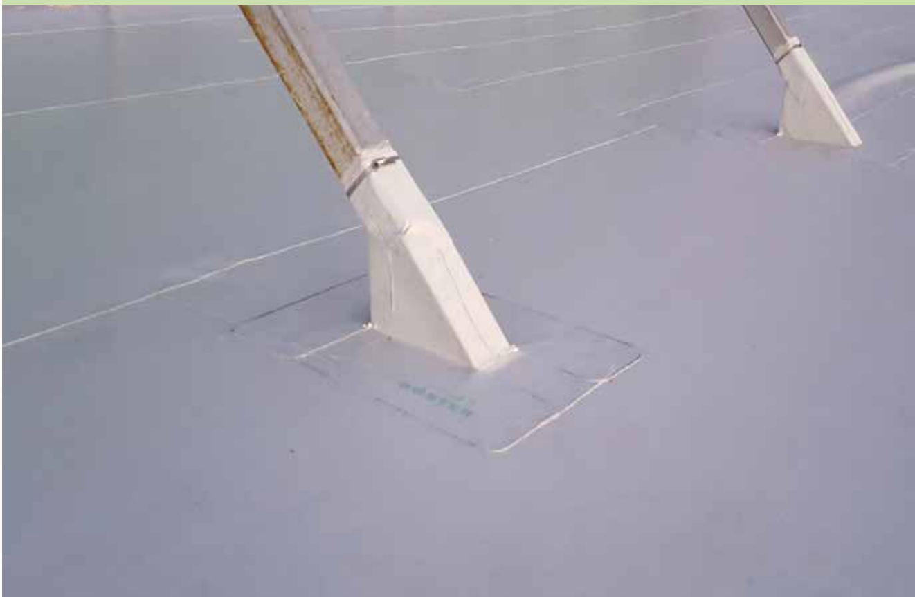
Junctions to right-angled penetrations
