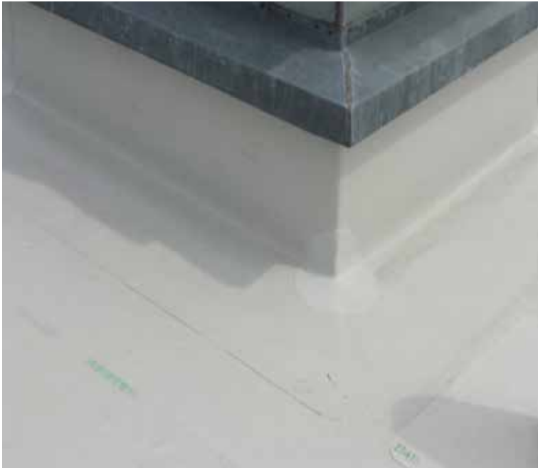
Junctions to right-angled penetrations
