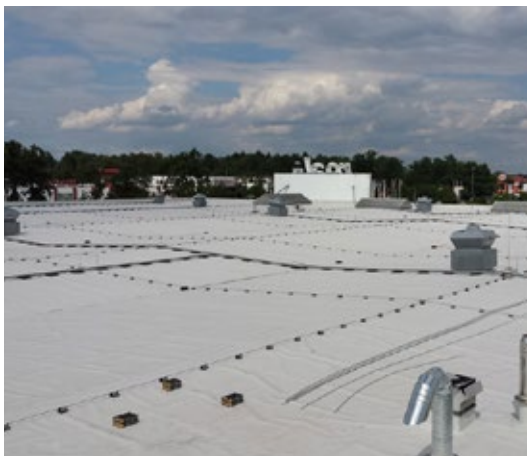
Flat roof waterproofing with KÖSTER TPO, REAL Supermarket, Germany
