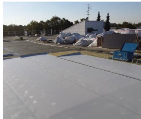
Flat roof waterproofing with KÖSTER TPO, EDEKA Supermarket, Germany
