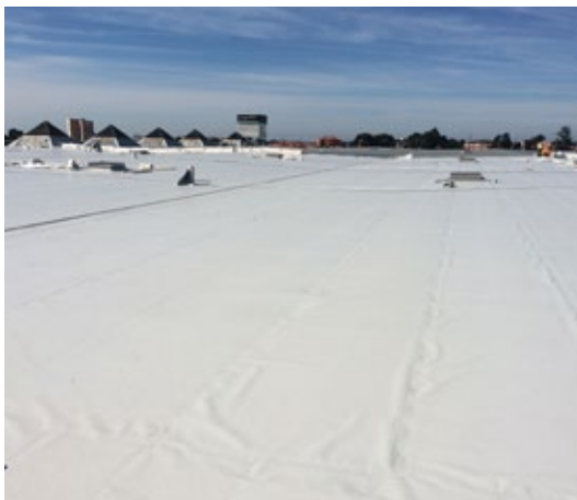
Flat roof waterproofing with KÖSTER TPO, Pingo Doce Supermarket, Portugal
